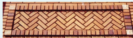
Herringbone brick pattern on former Bank of Toronto, in Assiniboia
